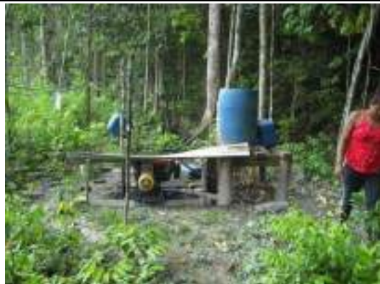
Foto 44: Motor – aldeia Lakariká (26/04/19).
